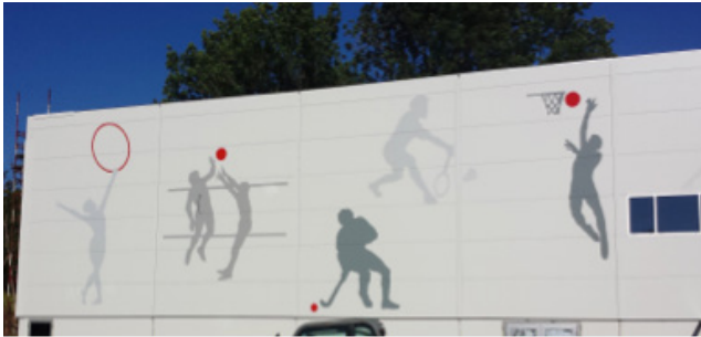
© Picture from the construction work. Ronnie Hollsten, Hifab AB
